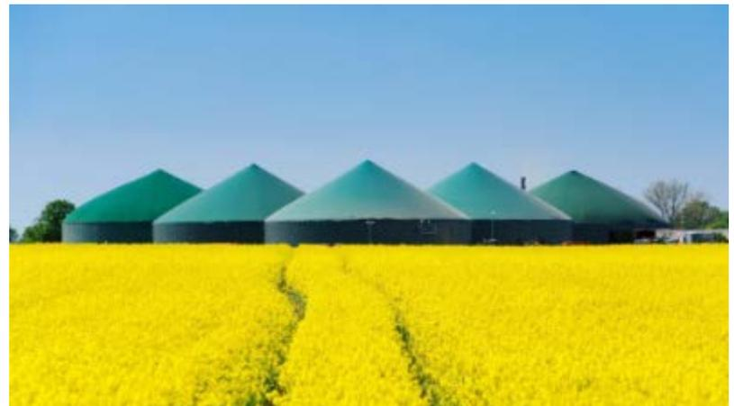
Biomass produced by manure, wood or organic waste can be turned into green gas through anaerobic digestion (already commercially available) or thermal gasification (not yet commercially available)
